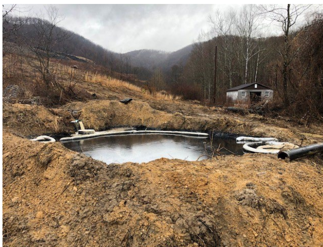
5 Retention downgradient from Outfall #3 impacted by pond overflow
