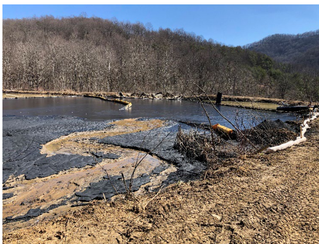
1 Heavy Sediment fills the pond to the surface on the south end
